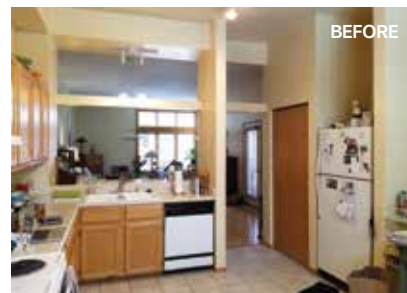
Prior to remodeling, finishes were dated and the refrigerator was tucked into a narrow alcove.
